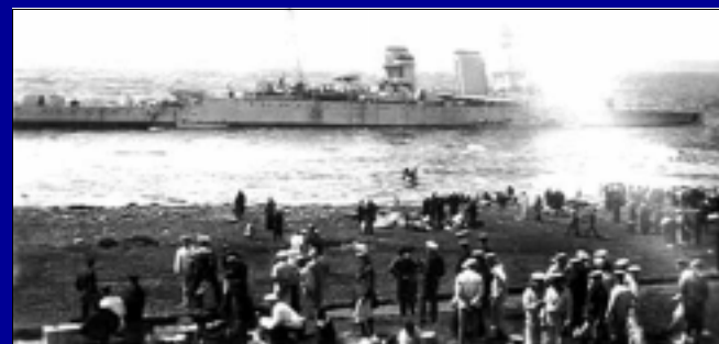
Raleigh aground, photograph probably taken on 9 August 1922, the day after the grounding, as the weather was bad on the 10th, and there were only a handful of her crew left at the scene in the days after.
